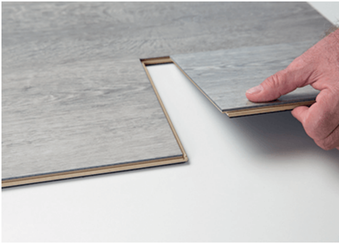
Start by engaging the plank on the long side (angle-system)
