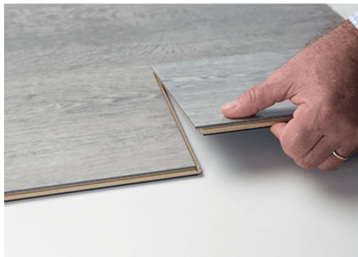
Slide the plank until it reaches the short side of the next plank.
