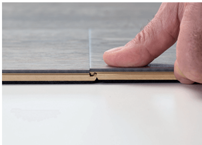
Press until you hear the “Click” sound of the drop-click-install system.
